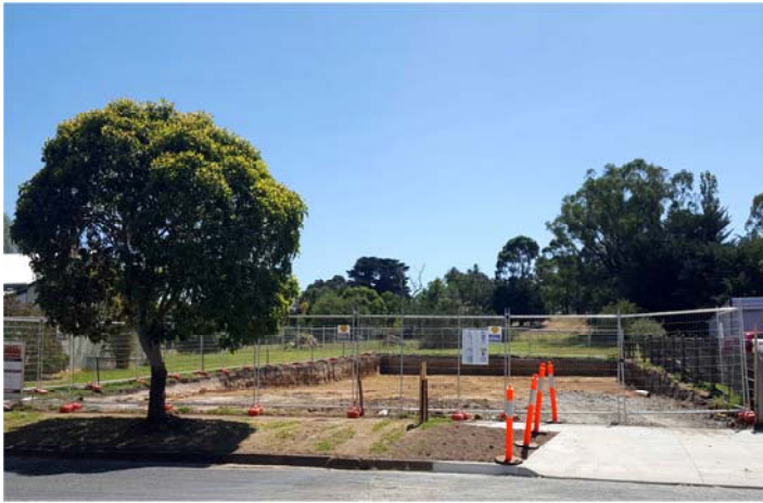
The site of the new Post Office prior to construction beginning.
